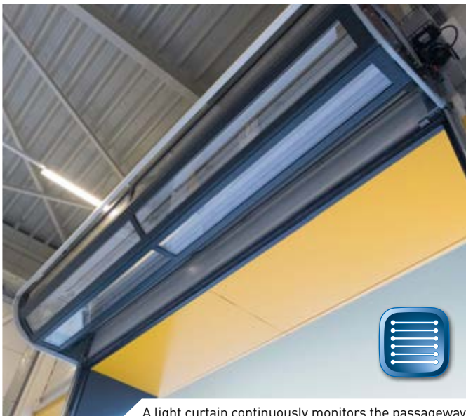
A light curtain continuously monitors the passageway
